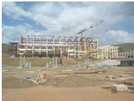
Olkaria II during construction
