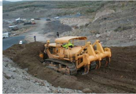
Minimal soil disturbance & rehabilitation
