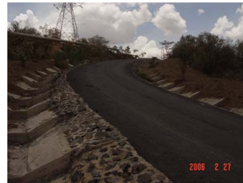
Road surface stabilized
