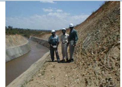
Soil erosion control
