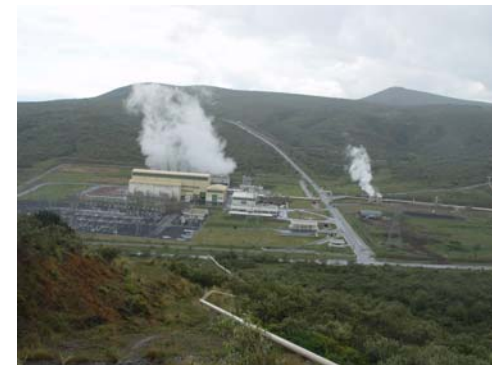
Olkaria II after construction
