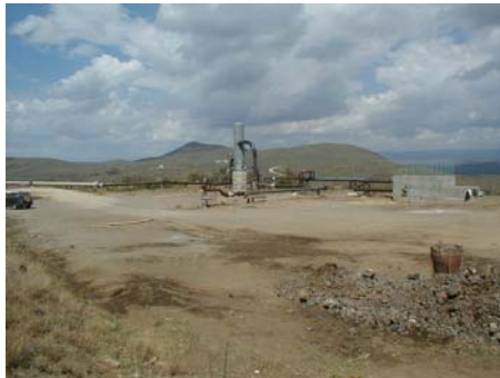
OW during works
